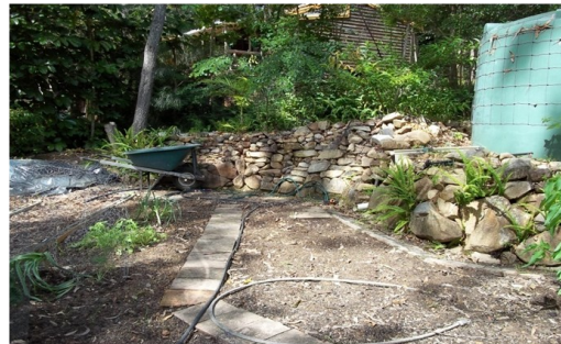
The hill cut away for the retainer wall, tank and vegetable garden
